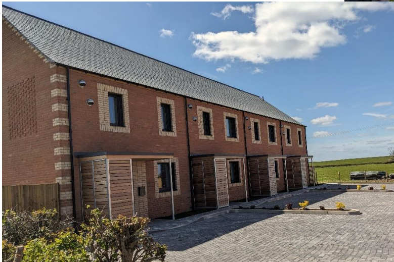
It's been a long time coming, but the first row of housing association super-energy-efficient homes in the Cleeve are ready. Don't they look smart?
